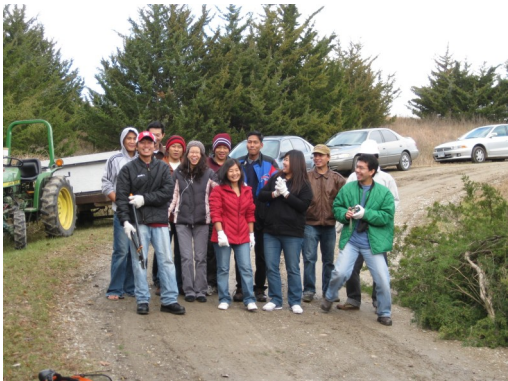
An energetic volunteer crew from First Kachin Baptist Church put in long hours on a recent Saturday. Another crew from Benson Baptist worked a long day and evening repairing the deck on Weaver
